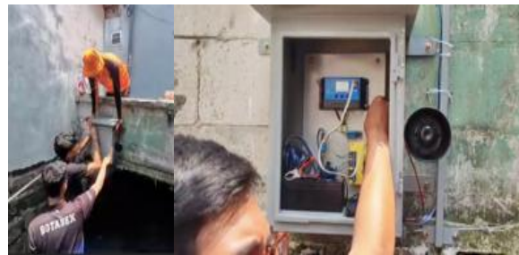
Fig 2. Installation of flood detection devices
