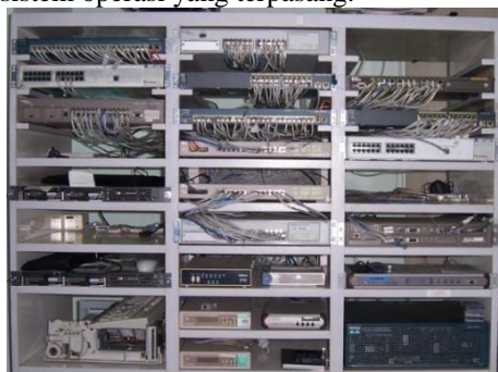
Gambar 11. Server PT. Bina Techindo Solution
