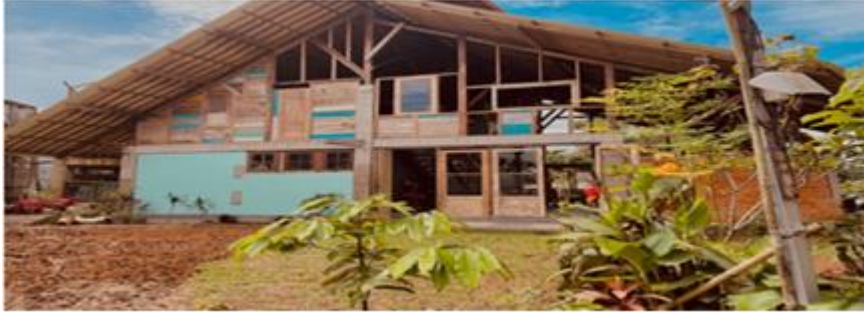
Figure.01: The New Misykat Al-Anwar School Building (source: researchers)
