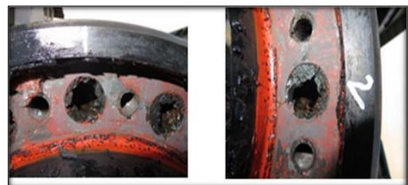
Fig. 8. Cooling water pipe hole
